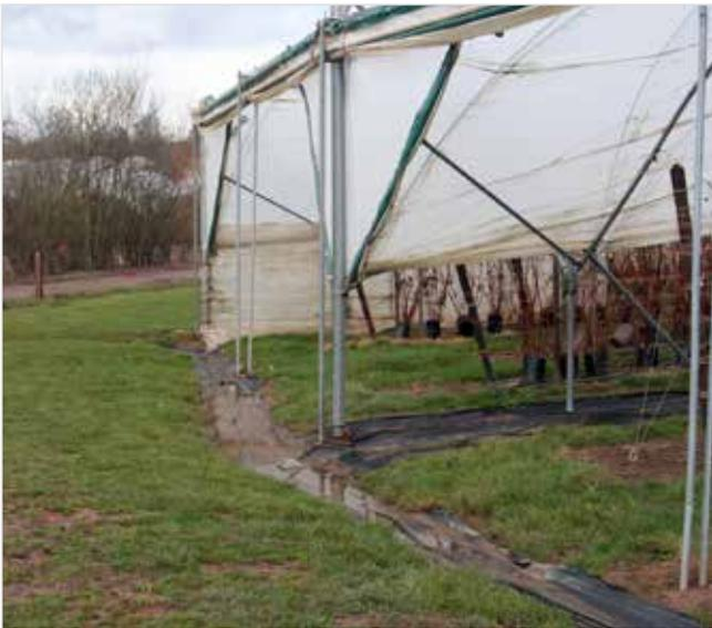
4. Shallow lined gullies to channel water from multi-bay tunnels not equipped with underground drainage pipes
