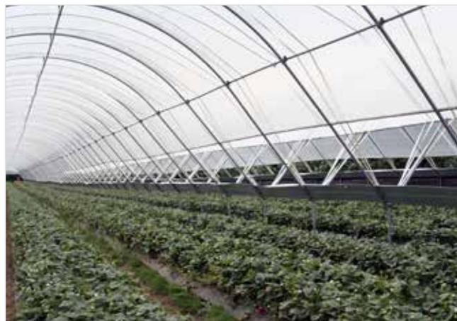
2. Gutter equipped multi-bay tunnel with automatic venting
