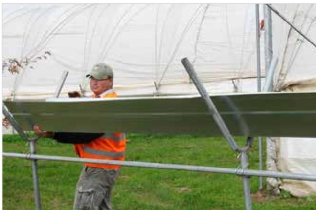
25. Metal gutters are cut and installed in Y-shaped legs to harvest rainwater between multi-bay tunnels
