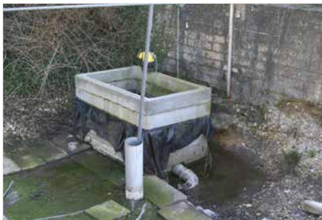
43. Silt trap prior to gravel bed
